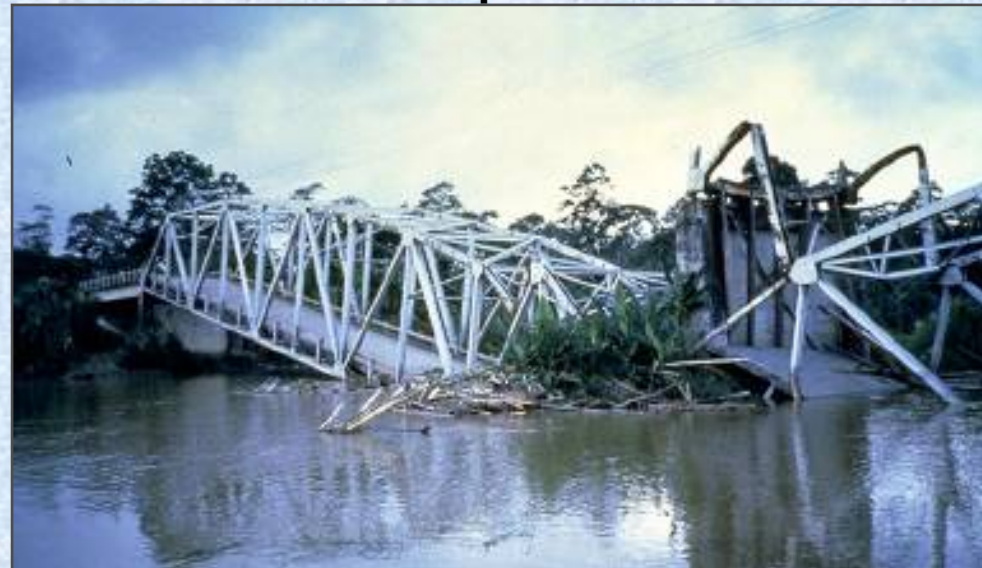
• Bridge failures during April 1991 M7.5 Costa Rica earthquake
